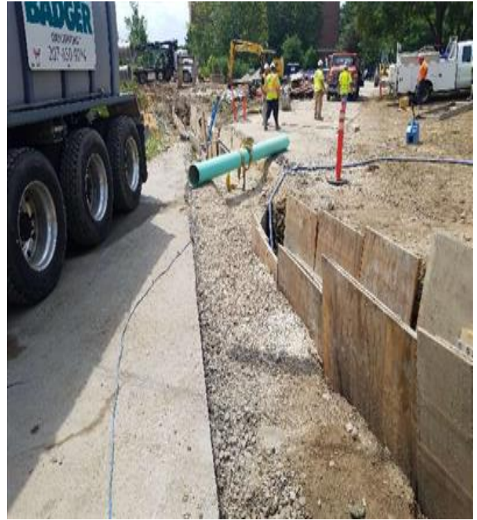
Fig 18: Trenching activities across Gregg Hall Rd. Viewing north. (8-07-19)
