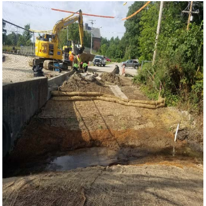
Fig 2: College Brook restoration. Viewing north. (8-01-19).
