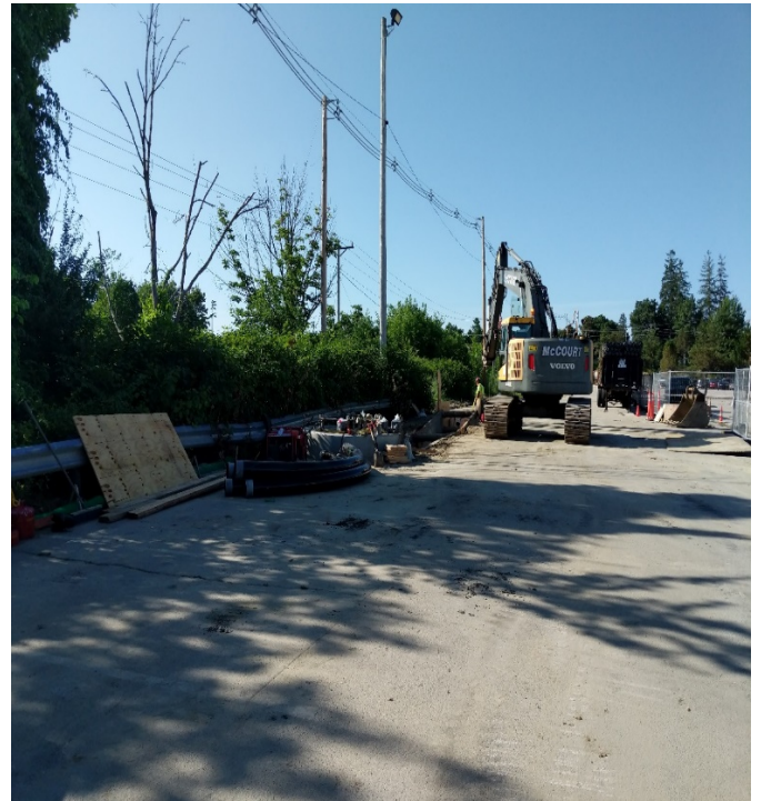
Fig 10: McCourt installing conduit for sweep to Str. 22. Viewing south. (8-05-19).
