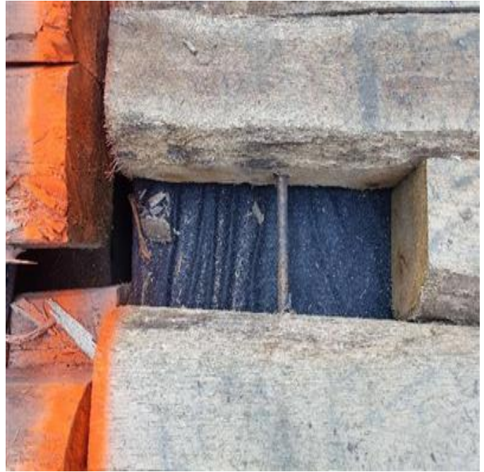
Fig 6: Filter fabric placed in between timber matting work pad for Str. 28. (8-02-19).
