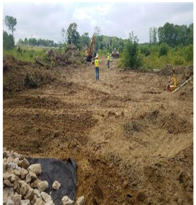
Fig 20: Constructing access road in the Shattuck laydown yard. Viewing west. (8-07-19)
