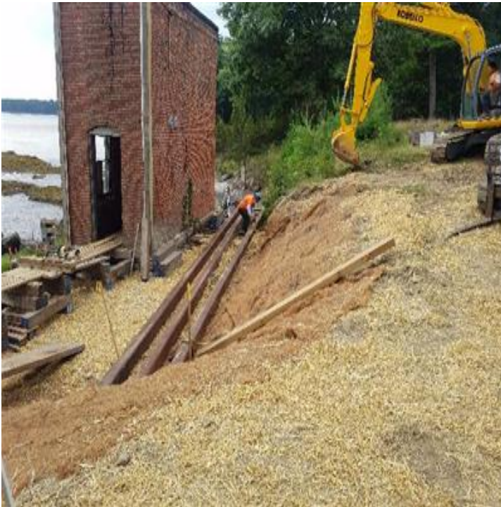
Fig 9: Gratan placing steel beams around the cable house. Viewing south. (8-03-19).
