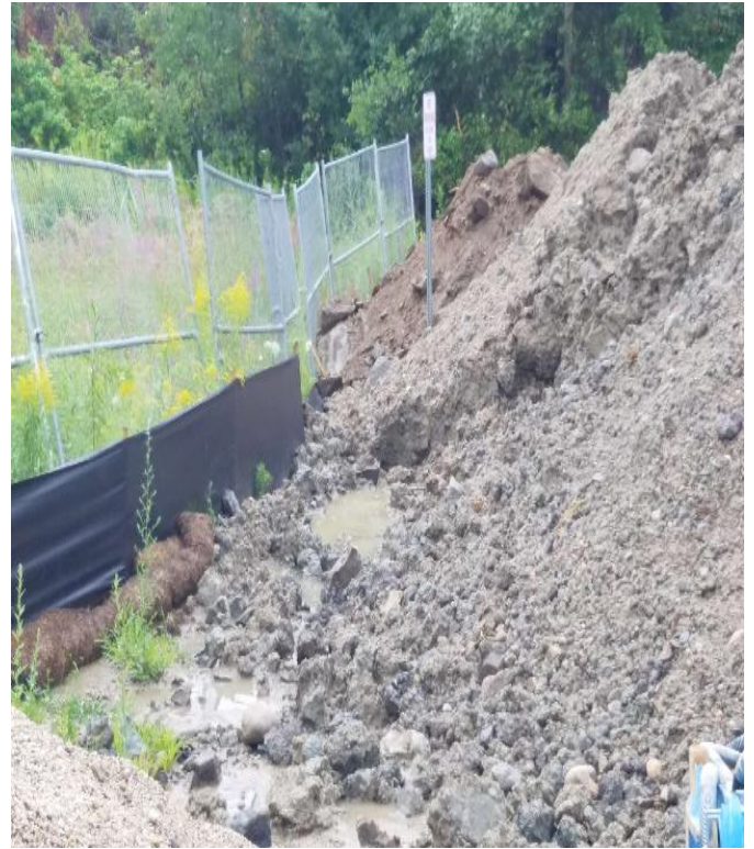
Fig 26: Waterworks Rd laydown yard. Viewing east. (8-08-19).
