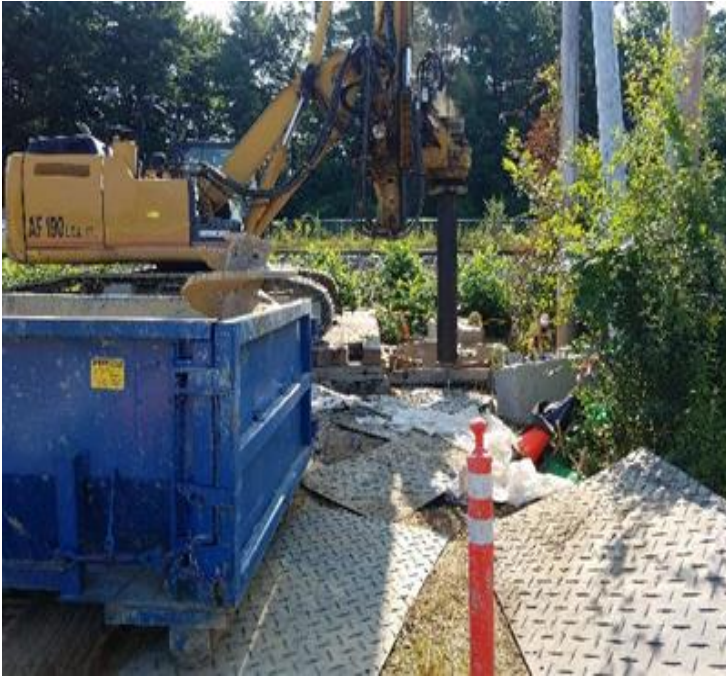
Fig 5: MJ drilling for Str. 21. Viewing east. (8-02-19).
