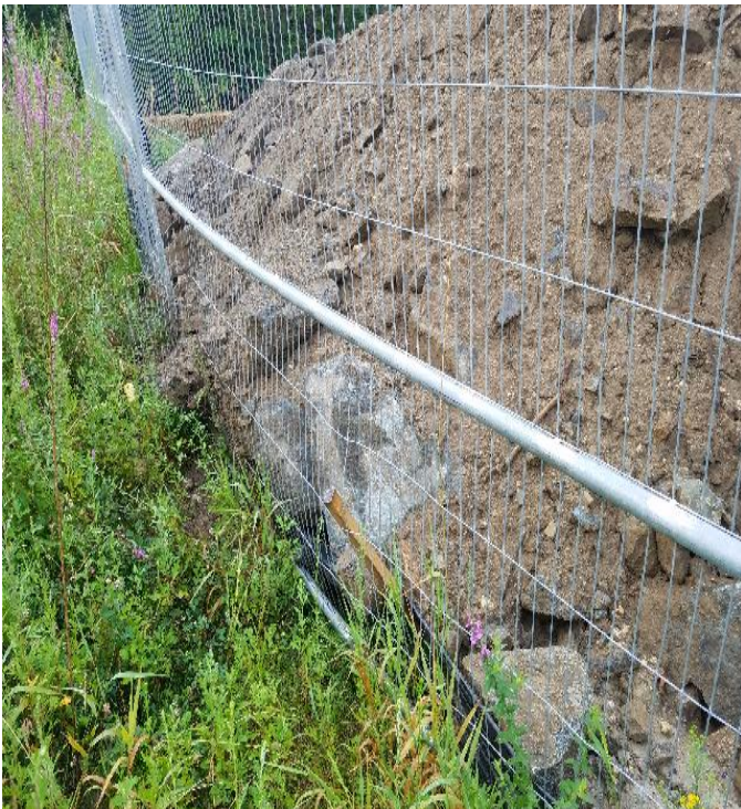
Fig 27: Waterworks Rd laydown yard. Viewing east. (8-08-19).
