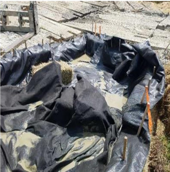
Fig 19: Newly built dewatering apparatus used for trench dewatering. Viewing south. (8-07-19).
