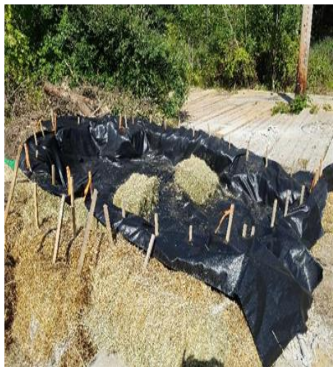
Fig 12: Dewatering apparatus installed near Str. 23 for McCourt's trenching activities. Viewing east. (8-05-19).
