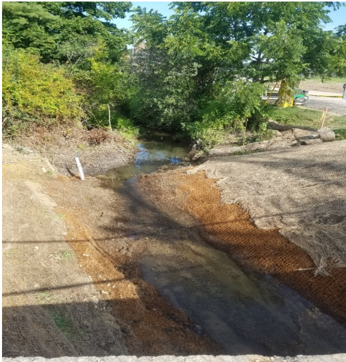
Fig 1: Upstream view of College Brook restoration. Viewing west. (8-01-19).
