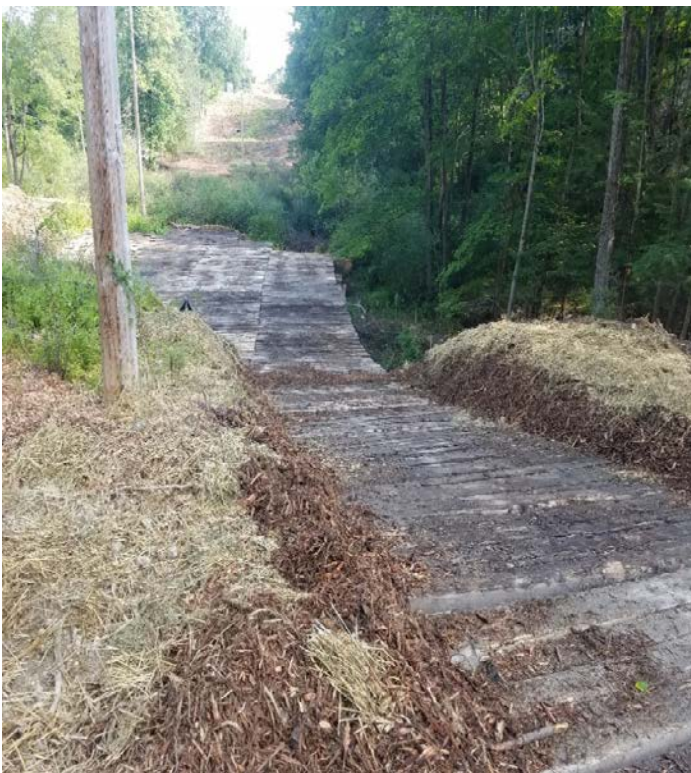
Fig 3: Wetland DW49 and work pad for Str. 28. Viewing north. (8-01-19)
