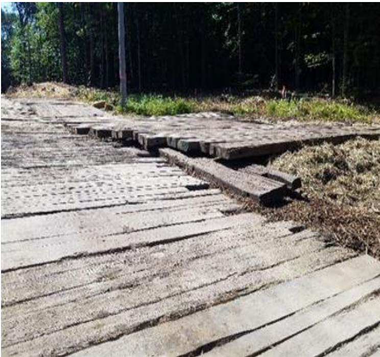
Fig 7: Work pad for Str. 29. Viewing south. (8-02-19).
