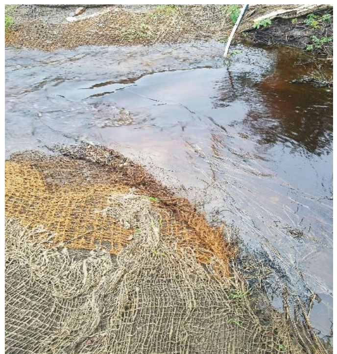
Fig 24: Restored section of College Brook. Viewing south. (8-8-19).
