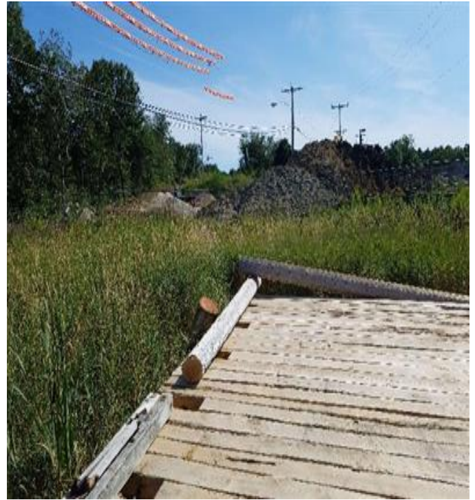
Fig 14: Existing structure in wetland DW65 removed. Viewing south. (8-05-19).
