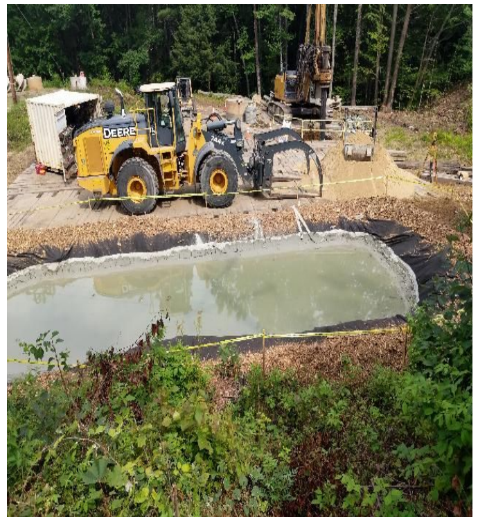
Fig 16: Dewatering basin next to drilling activities at Str. 32. Viewing east. (8-06-19).
